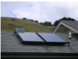
M.7 Install Solar Water Heating System
